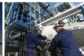
Heating & cooling Systems & Pipework
